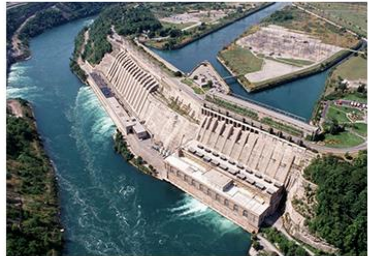
Hydroelectric plant generating power from the energy of rushing water
